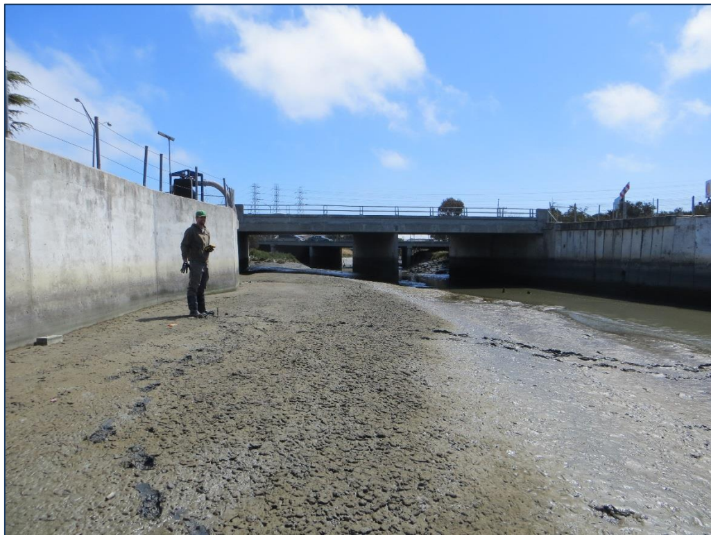
Photo 6: A large point bar in Reach 2c (looking downstream toward Produce Ave).
