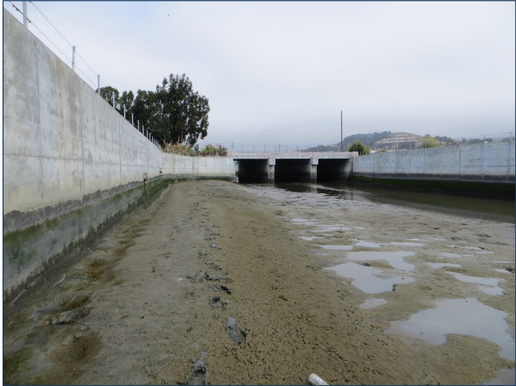
Photo 5: Reach 2b looking upstream at the Caltrain railroad bridge. Sediment deposits downstream of the bridge on the left side of the photo, where flow separation and eddying create a depositional environment.
