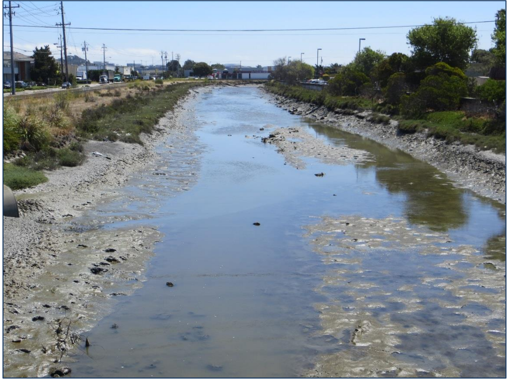
Photo 7: Reach 3 looking downstream from Produce Avenue at low tide. Note earthen bed and banks comprised of fine sediment, some depositional bars along channel bed, and mid-bank bench with pickleweed.
